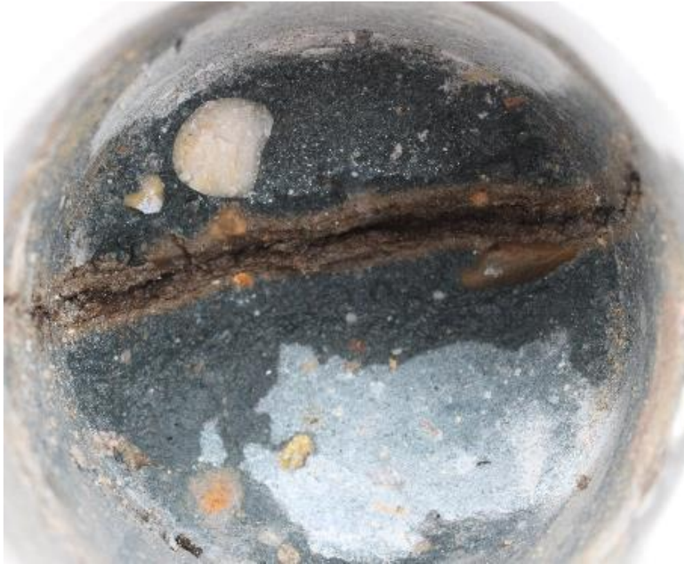
Crack in concrete substrate
