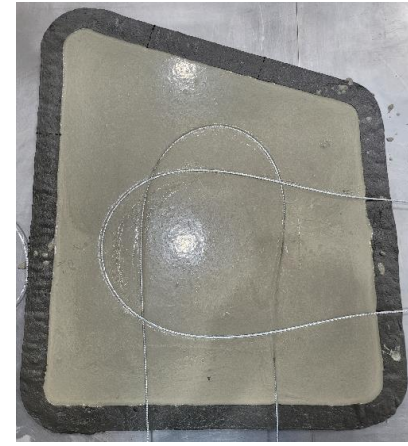
Step 3: Placing cable
