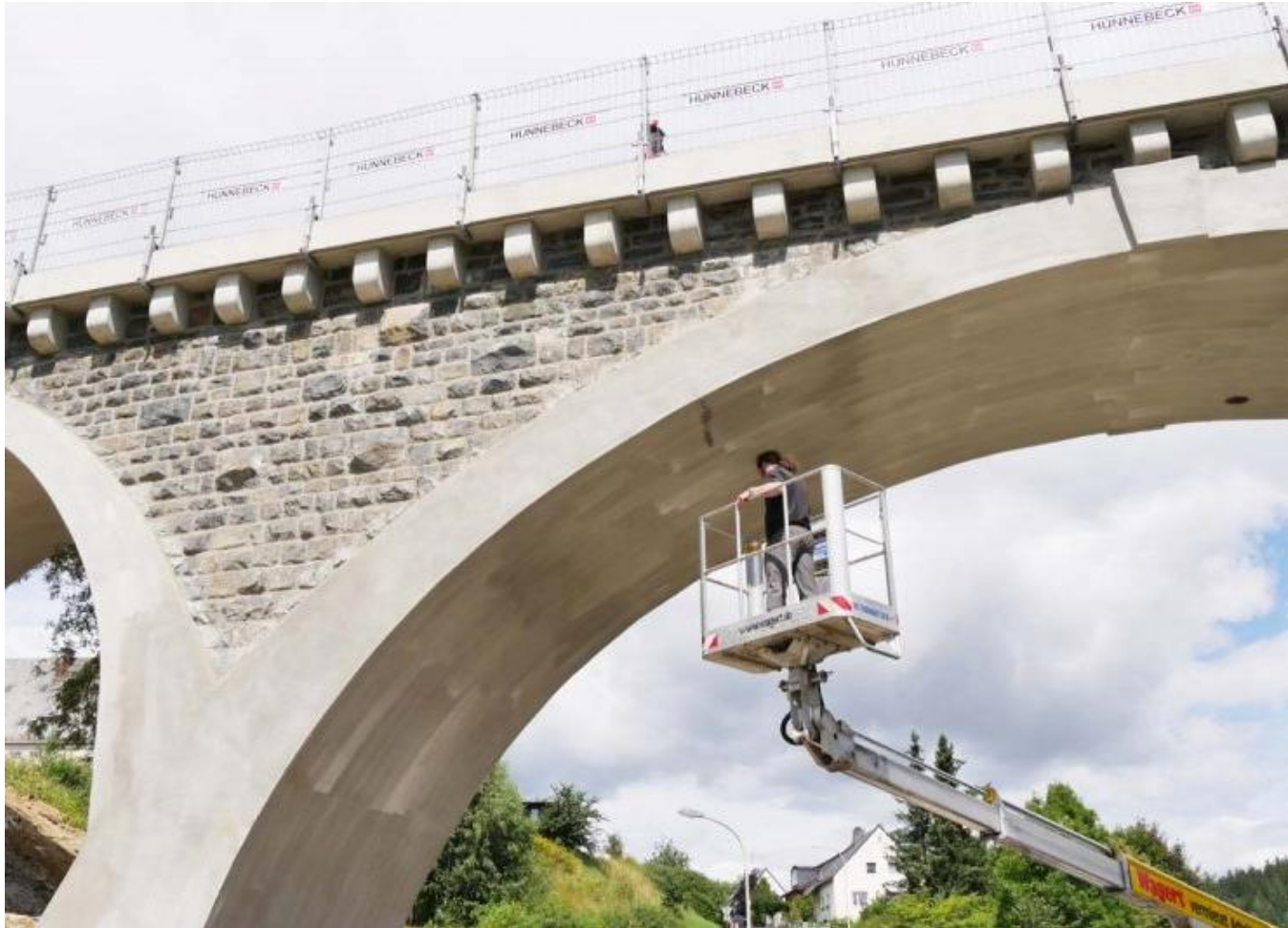
Strengthening / Repair / Rehabilitation
